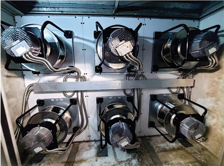
◀ AHU Replacement of EC Plug Fans
